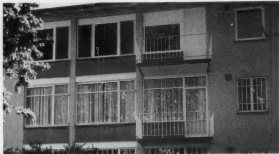
In the Bonn housing complex, first and second floors have the original steel-framed
